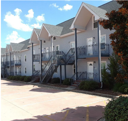
Georgia Southern University Siding
