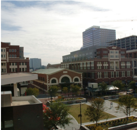
Atlantic Station Condo, Chilled Water Replacement
