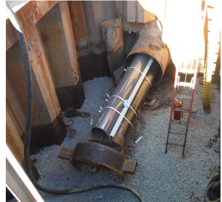
Baltimore Food Hub IMTT Galvanic CP System for 48" Steel Casing Pipe
