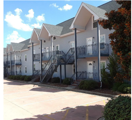
Georgia Southern University Siding
