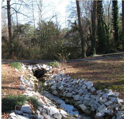
DeKalb County Stormwater Upgrade
