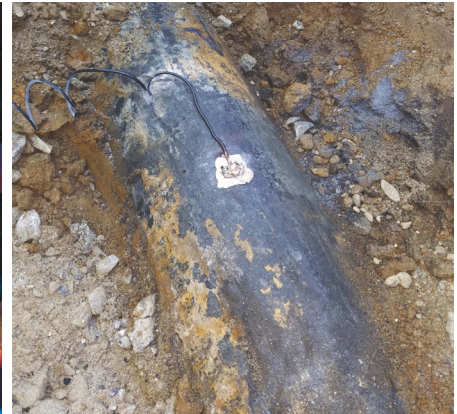
Wilde Lake, Water Main Study & Rehabilitation
