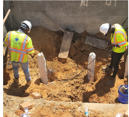
DC Water Anode Installation, Washington DC
