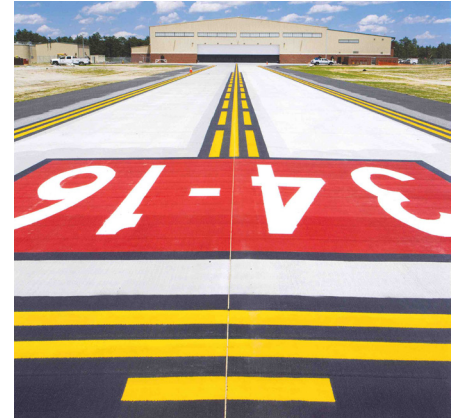
Unmanned Aerial Vehicle (UAV) Hangar & Runway
