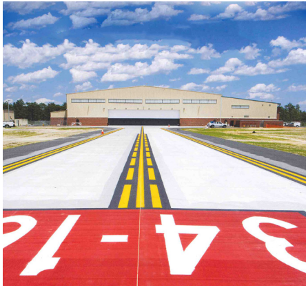
Unmanned Aircraft Vehicle Hangar (UAV)
