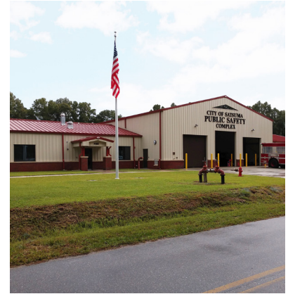
Satsuma Public Safety Building
