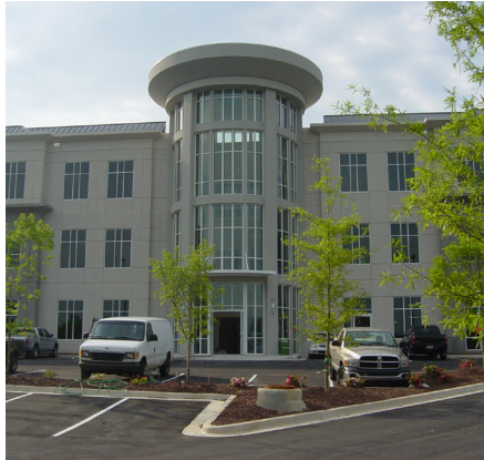
Hillandale Medical Office Building
