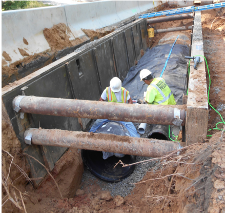
North Area Water Main Replacement, Section 2
