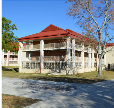
TBUP Barracks Renovations
