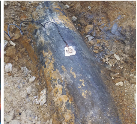
Wilde Lake, Water Main Study & Rehabilitation
