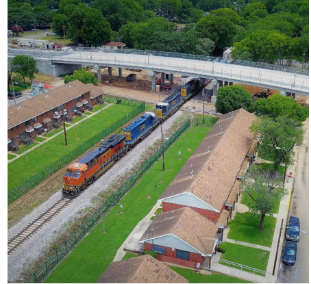
Shuttlesworth Bridge, Birmingham
