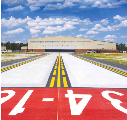
Unmanned Aircraft Vehicle Hangar (UAV)
